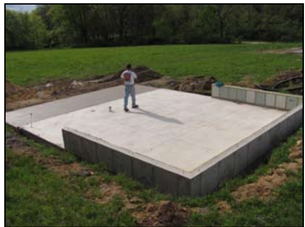
Concrete floors and foundations were poured in May as work began on two sustainable living cabins at Fontana Park.
