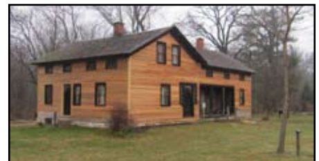
New siding on the "Old House" will be stained red this spring.
