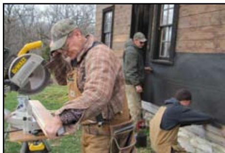
Above: Conservation Volunteer Don Shonka cuts siding boards to length, as others nail boards in place.
